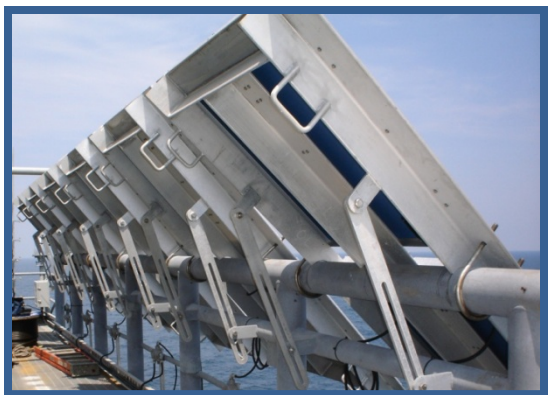
Chevron ESS System Eastern GOM
