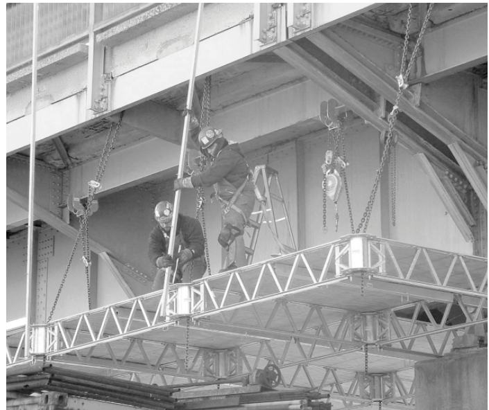
Workers attaching Integral Railing and Containment Post.
